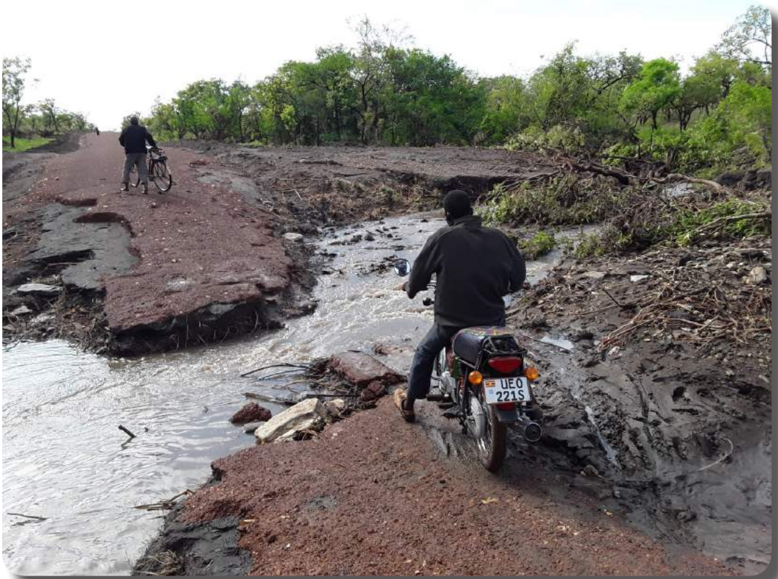
In Palabek Ogili, one heavy rainfall washed away a newly constructed road overnight, preventing the screening team from accessing the site
